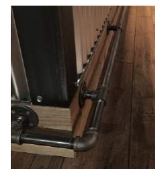
Gas pipe kick bar mounted to floor
